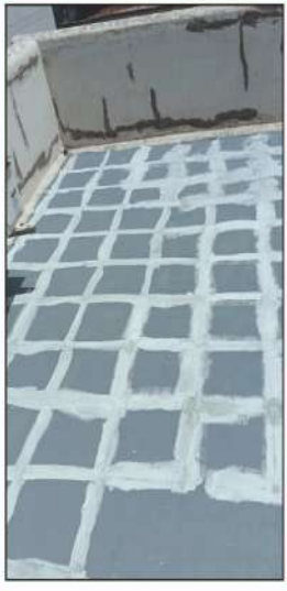
Bhujpur Terrace Before Work
