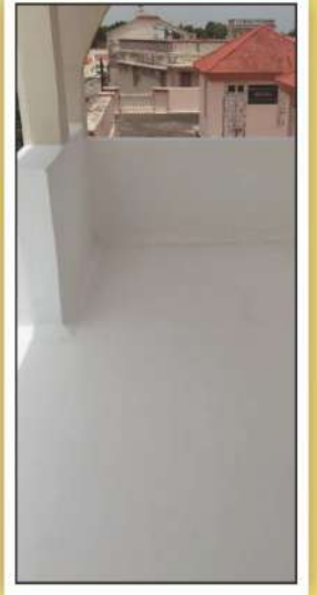
Bhujpur Terrace After Work
